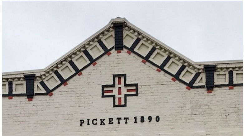
Figure 11. The building parapet retains its brick work details.
