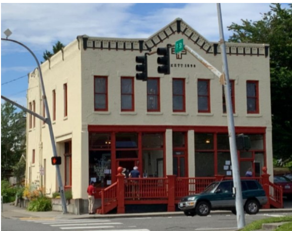
Figure 10. Oblique view of the building showing the Dupont and F Street facades.
