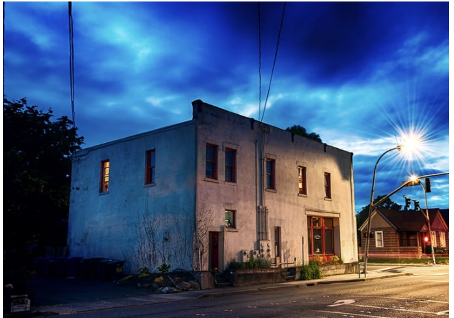
Figure 13. 2016 photo of the building by Patrick Beqqan, Flickr.
