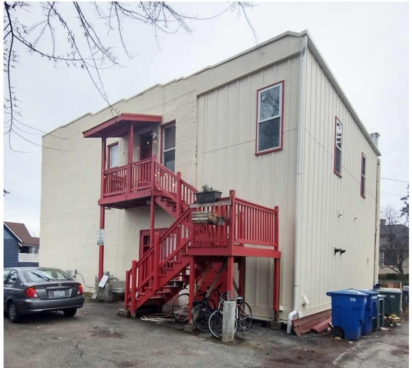
Figure 18. Northwestern side and southwestern rear facades of the building.
