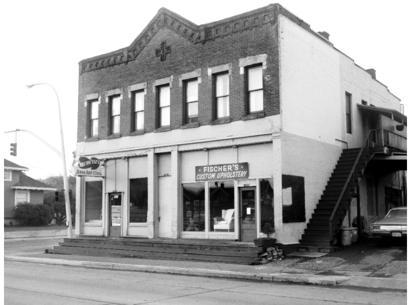
Figure 9. Historic photo of the Dupont Street facade, showing Fischer's Custom Upholstery, 1971. Photo by Galen Biery, courtesy Whatcom Museum.
