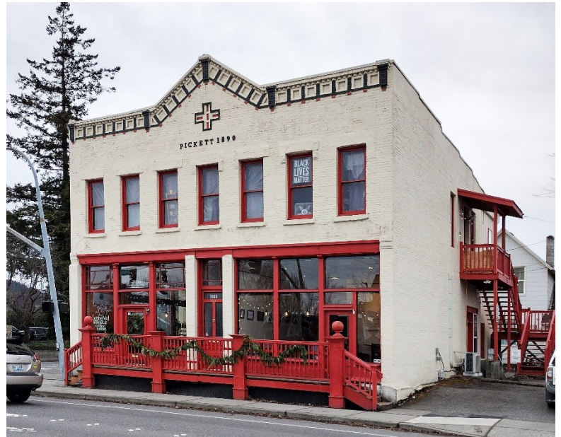
Figure 8. Current photo of the northeast primary façade, fronting on Dupont Street.
