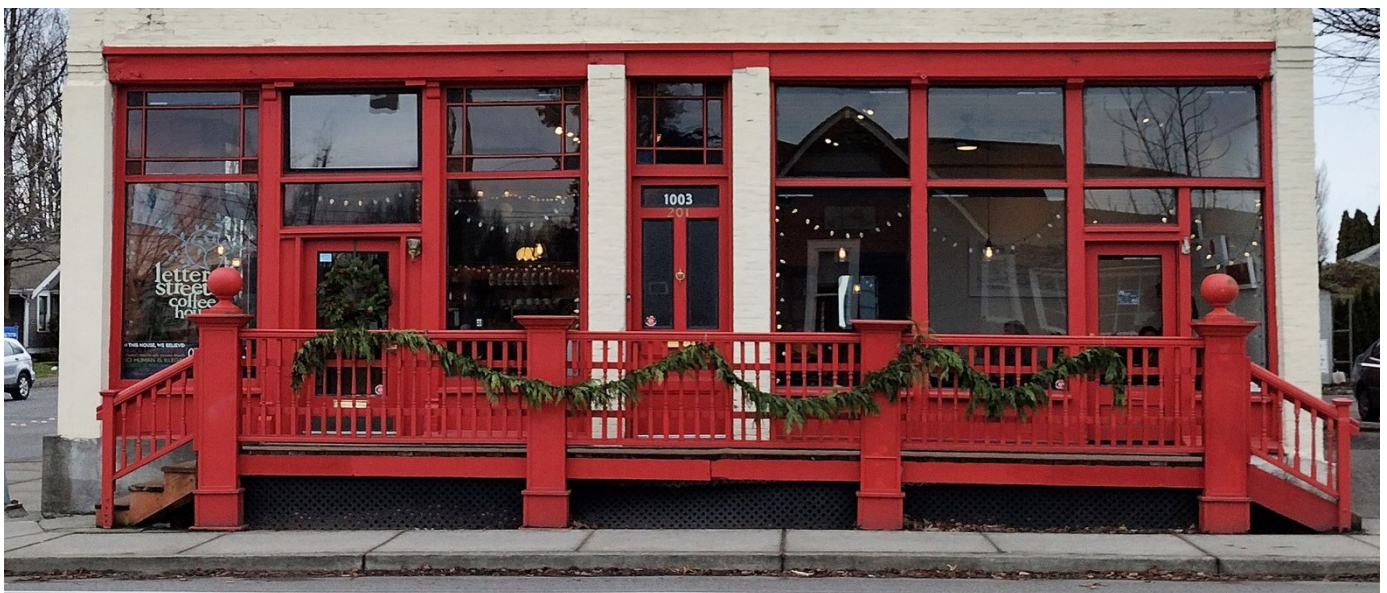
Figure 12. The main façade has a symmetrical layout to the commercial spaces, flanking the centrally located stairway door. It appears that three divided light transom windows remain intact, two on the eastern space and one over the upper story door. The western commercial windows are not symmetrical, suggesting that the entry door may have originally been located within the center window opening.
