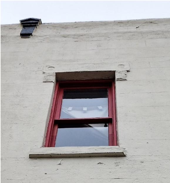
Figure 14. The F Street façade has had stucco applied over the brick and a faint faux block pattern traced into the stucco. Some of the original detail of the lintel, the lintel bracket, and the decorative bullseye remain.
