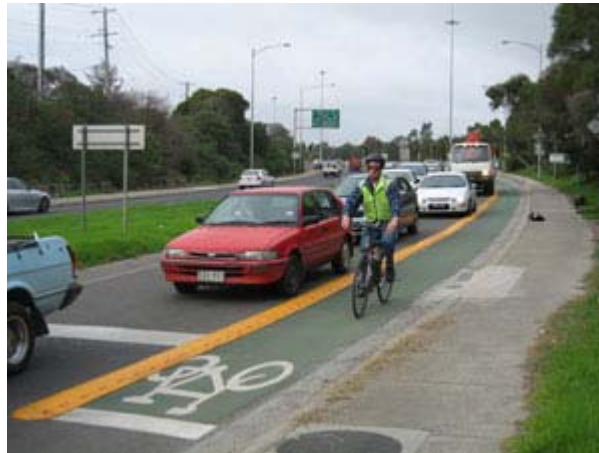
Figure 3: Separator installed along Chandler Highway.
