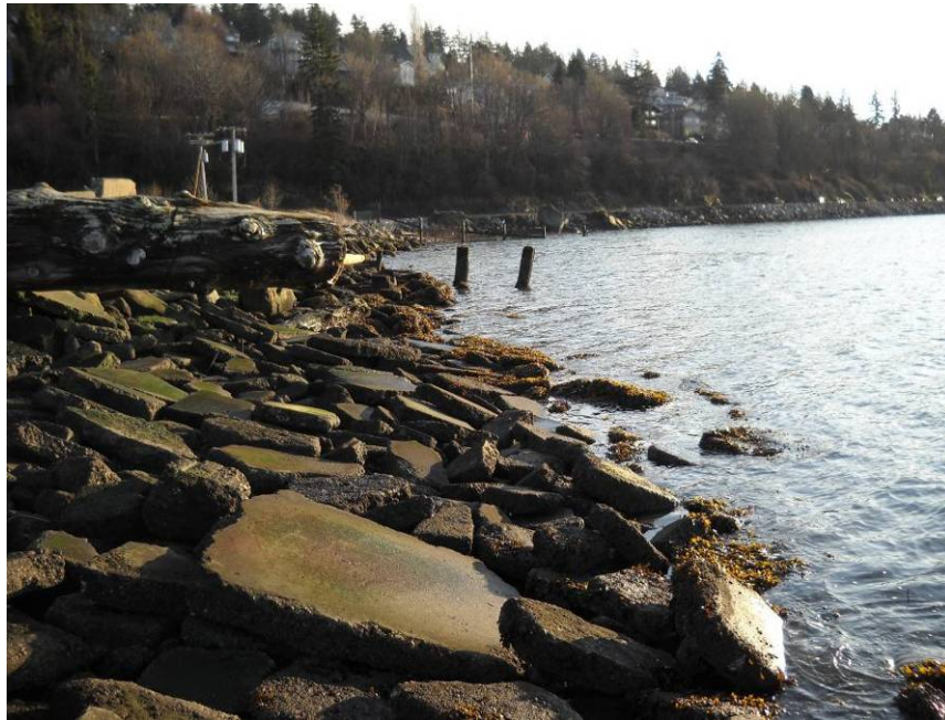
Photo 3 – View of the former Cornwall Avenue Landfill site where the north abutment of the proposed overwater walkway will land (facing southeast)
