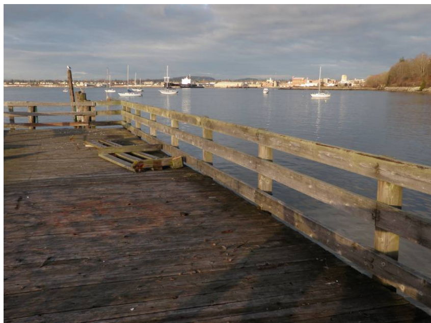
Photo 4 – View of proposed overwater walkway location from the existing pier at Boulevard Park where the southern end of the walkway will land (facing northeast)
