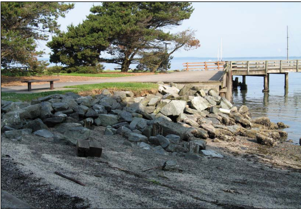
Figure 4 The vicinity of the southern abutment location in the Boulevard/Cornwall Overwater Pedestrian Walkway Project Area. The abutment will be located where the pier meets the wharf in the middle distance. View is to the northwest.
