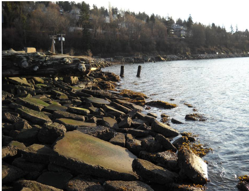
Photo 3 – View of the former Cornwall Avenue Landfill site where the north abutment of the proposed overwater walkway will land (facing southeast)
