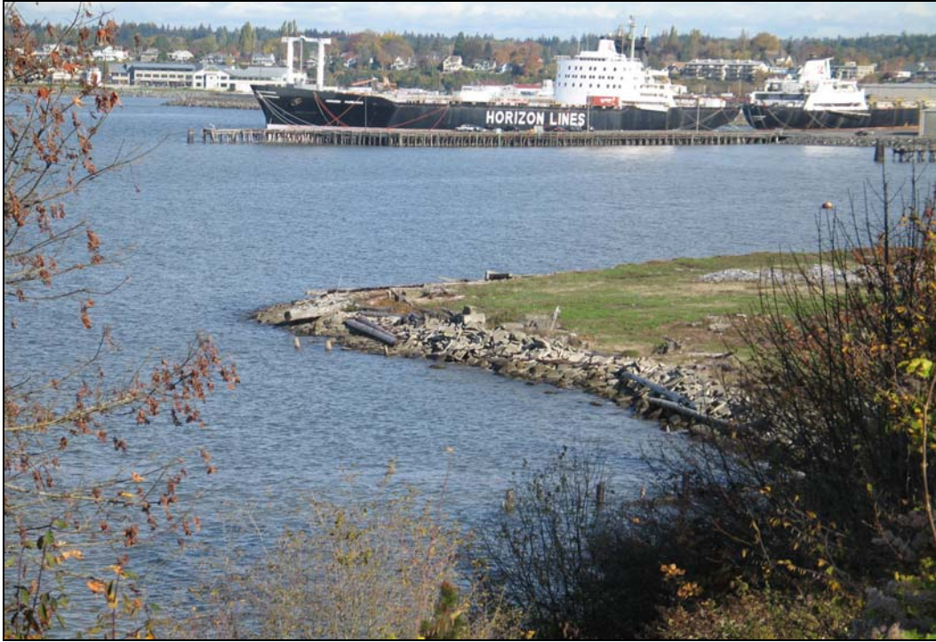
Figure 5 An overview of the vicinity of the northern abutment location in the Boulevard/Cornwall Overwater Pedestrian Walkway Project Area. View is to the north.
