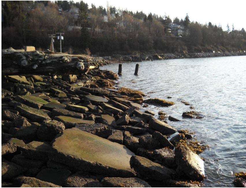
Photo 3 – View of the former Cornwall Avenue Landfill site where the north abutment of the proposed overwater walkway will land (facing southeast)
