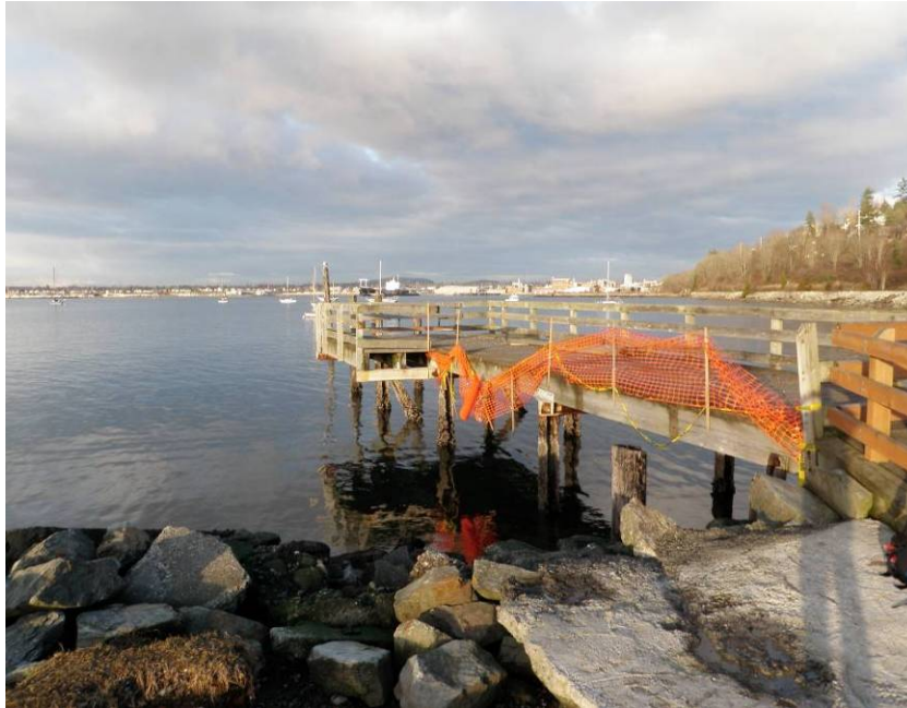
Photo 2 – View from Boulevard Park of the existing pier where the southern end of the overwater walkway will land (facing north)
