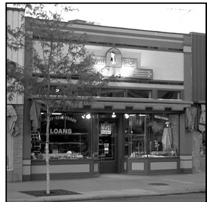
The same building (above) after renovation, exhibits the more classical features of commercial storefronts, including a painted cornice, kickplate, and recessed entry.
