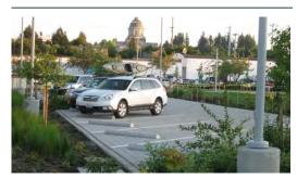
Pervious paving and raingarden stormwater treatment at Percival Landing in Olympia (Photo: Anchor QEA)
