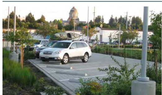
Pervious paving and raingarden stormwater treatment at Percival Landing in Olympia (Photo: Anchor QEA)
