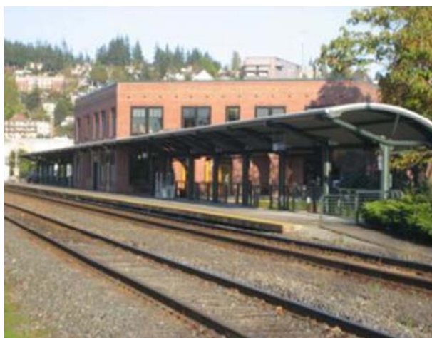
Figure 33: Looking northeast along Burlington Northern Railroad tracks to Bellingham Station.
