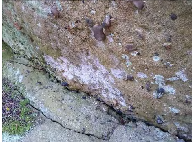
Photo 10: Conglomerate Bedrock Exposure; SW Project Area
