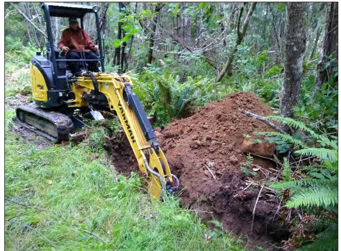
Photo 4: TP8 Location; Excavated Glacial Drift
