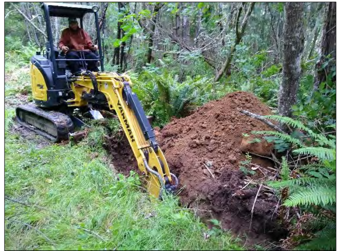
Photo 4: TP8 Location; Excavated Glacial Drift
