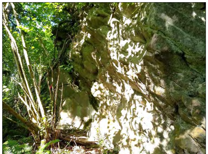
Photo 6: Central Area of NW Bedrock Face
