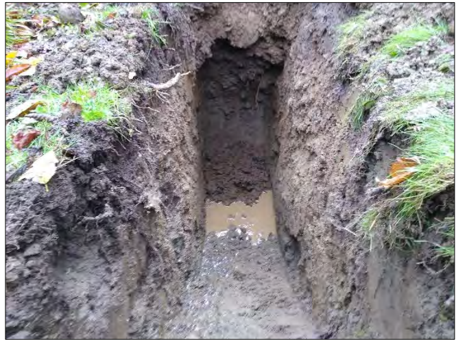
Photo 4: TP2 Caving on South Pit-Wall
