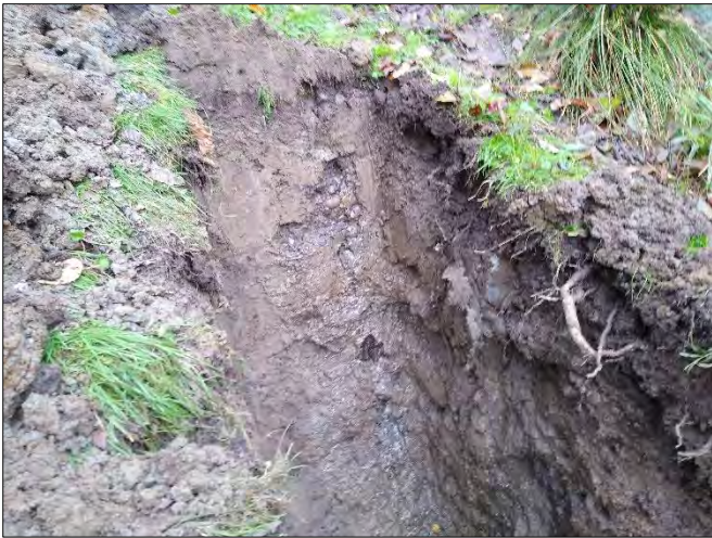
Photo 3: TP2 Seepage from North Pit-Wall
