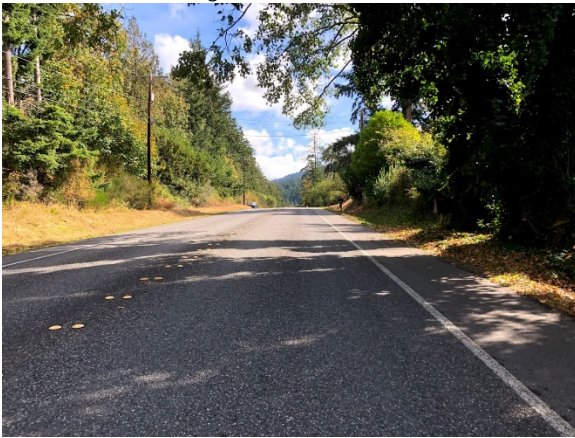
View looking South approaching Viewcrest Rd
