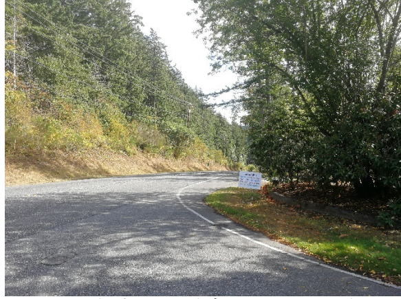
View looking South from Viewcrest Rd
