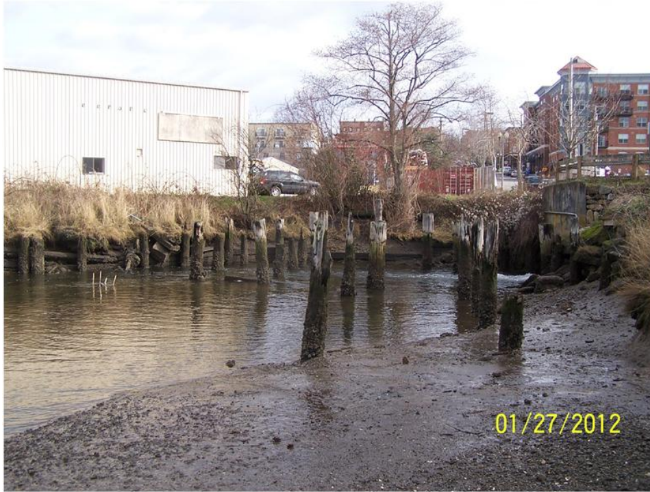
Figure 15. Photo of bulkhead and pilings in the southeast corner of the subject property (above) and urban trash in middle of estuary (below).
