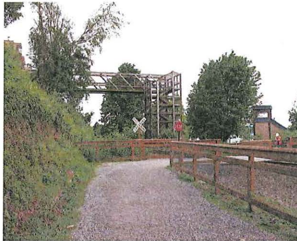
Figure 9 - Boulevard Park Pedestrian path facing west. Pedestrian crossing crosses tracks to the right of the stop sign shown.
