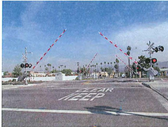
Figure 1 – Four-Quadrant Gate System
