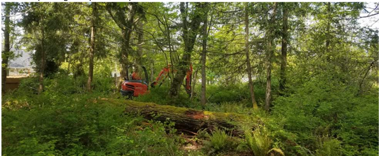
Image 1 – Typical surface conditions of site interior. View facing north with test pit TP-9 in progress.
