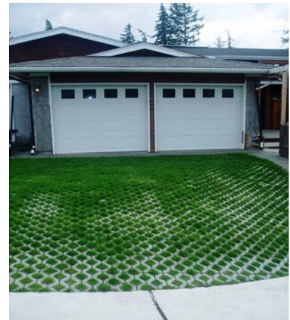
Pervious driveway in Lake Whatcom Watershed
