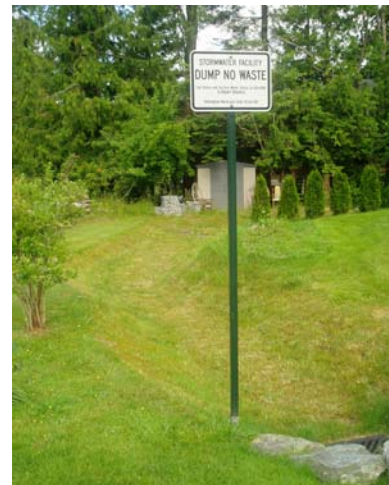
Maynard infiltration swale
