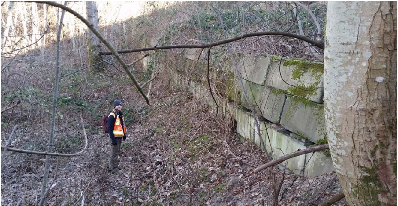
Photo C: View facing NE at ecology block wall. Note deformation and improvised repairs at the top of the second lift of blocks. First course of blocks is mostly obscured by soils and vegetation.
