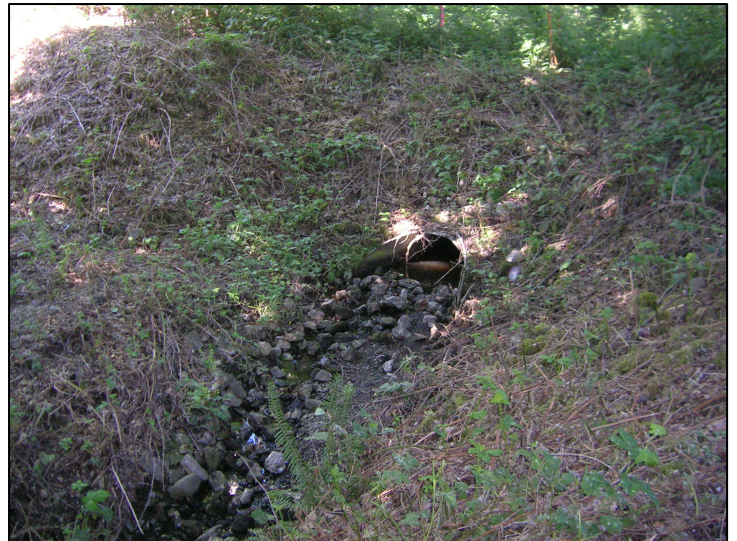
Birchwood Neighborhood/Bellingham Technical College stormsewer outfall as seen facing north (June 2009).
