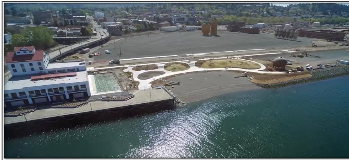
Photo of Granary Building and Waypoint Park along Whatcom Waterway
