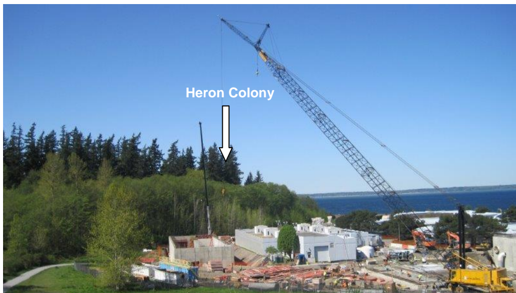
Post Point Wastewater Plant expansion 4.25.2013
