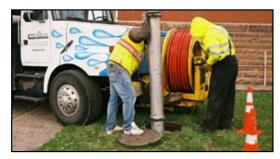
Wet vaults are large underground storage tanks that use settling for pollutant removal. Periodic inspection of control structures is needed. Typical maintenance requires the use of a vactor truck.
