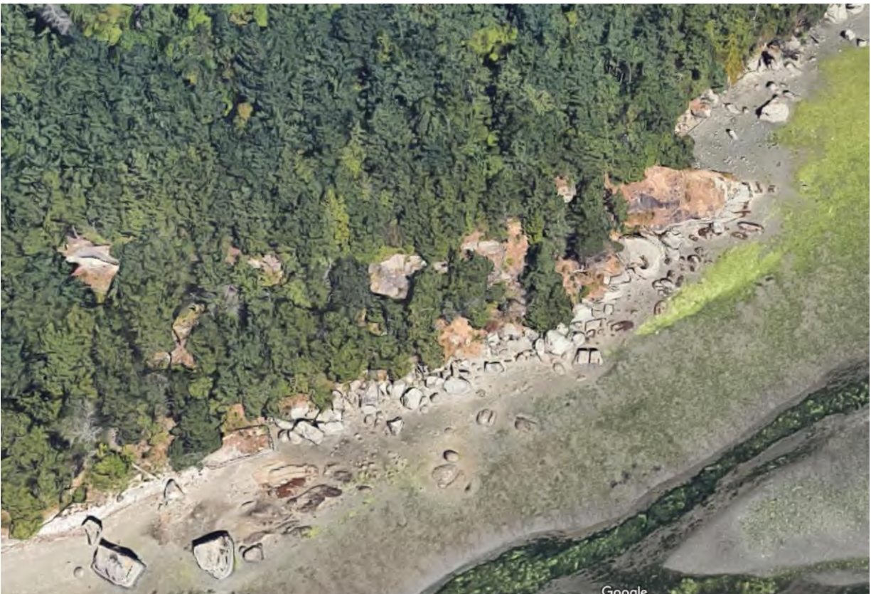
Figure 4. Evidence of rock fall along the southern boundary of the property.
