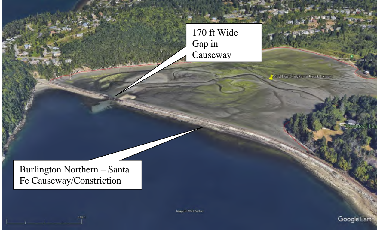
Figure 6. The Burlington Northern – Santa Fe Trestle at the Southern End of Mud Bay. [Source – Google Earth Image May 16, 2023]
