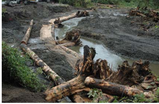
Second layer of LWD.
