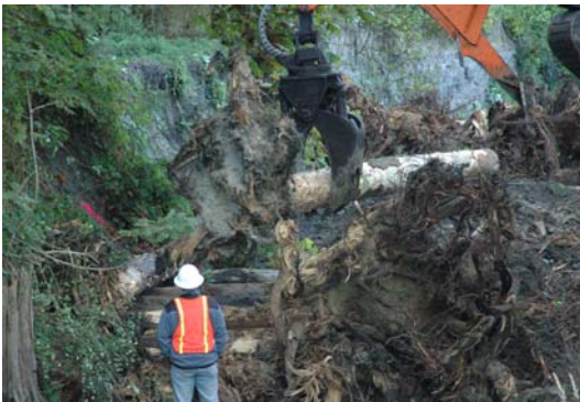
LWD placement in left bank.
