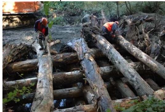
Drilling holes in LWD to cable wood.
