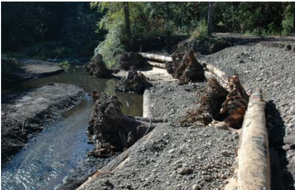
Completed LWD installment, looking downstream.
