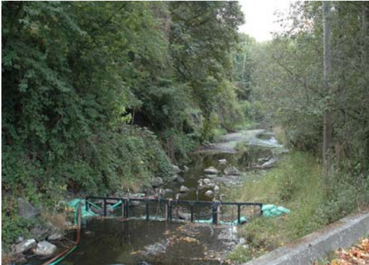
Fish screening installed prior to construction.
