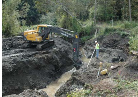
Heavy machinery creates notches for LWD that will help redirect streamflow.
