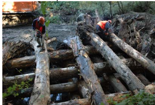
Drilling holes in LWD to cable wood.
