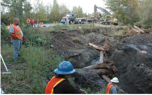
LWD structures embedded in right bank.
