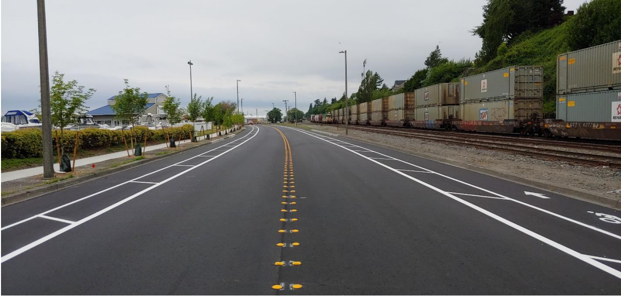
Roeder Avenue in May 2019 – Resurfaced; Rechanelized with Buffer-Separated Bike Lanes; On-street parking removed, but possibility for accommodation of parking for major community events, such as Ski to Sea Race; July 4 th ; SeaFeast; Bellingham Bay Marathon; etc.
