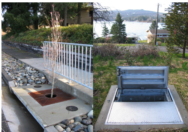
Figure 4.0-1. Bellingham is leading the way in stormwater treatment by installing the new Filterra™ vault (left) and Alumina filter media vault (right) in the Lake Whatcom watershed.
