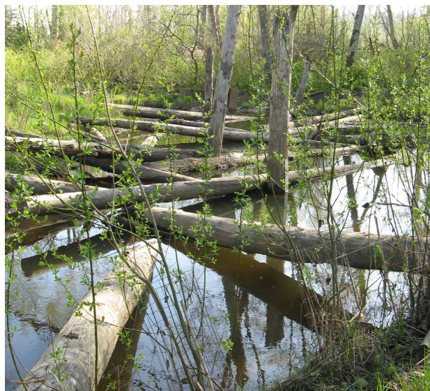
Figure 2.0-4. Backwater pond created on Cemetery Creek to provide low velocity refuge for juvenile fish in times of high flow.
