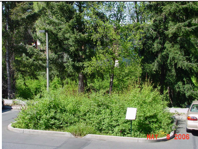
Figure 4.0-2. Rain garden in the Bellingham City Hall parking lot. Run-off enters the rain garden through the curb cut shown in the photograph. Pollutants are taken up by the plants or removed by filtration within the soils. Treated water is slowly discharged to Whatcom Creek, behind the rain garden.
