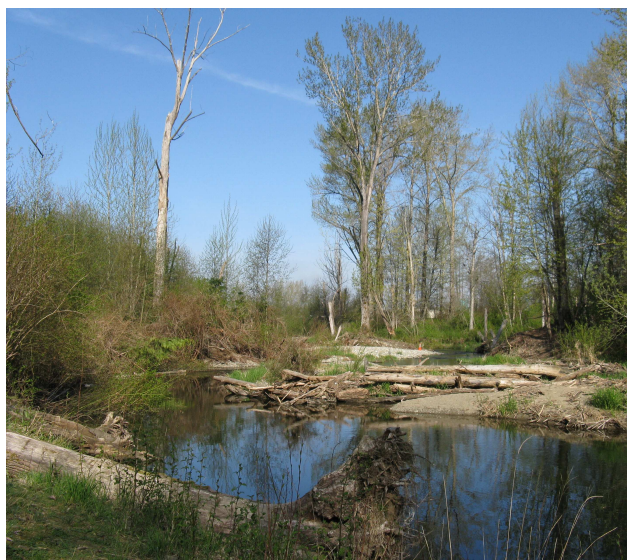
Figure 2.0-3. Placement of root wads and large woody debris for bank stabilization on Whatcom Creek.
