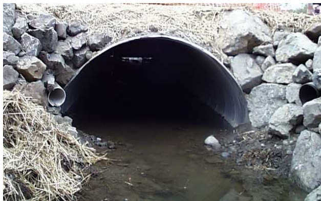
Figure 2.0-2. Fish-passable culvert on Connelly Creek at Donovan Ave.
