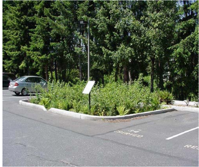
Figure 4.0-2. Rain garden in the Bellingham City Hall parking lot. Run-off enters the rain garden through the curb cut shown in the photograph. Pollutants are taken up by the plants or removed by filtration within the soils. Treated water is slowly discharged to Whatcom Creek, behind the rain garden.
