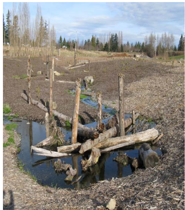
Figure 3.1-1. Daylighted area of Willow Spring. Depicted in the foreground is the newly created winding course and instream large woody debris.
