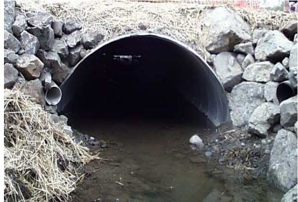
Figure 2.0-1. Fish-passable culvert on Connelly Creek at Donovan Ave.
