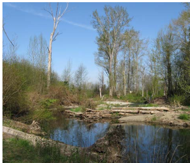
Figure 2.0-2. Placement of root wads and large woody debris for bank stabilization on Whatcom Creek.
