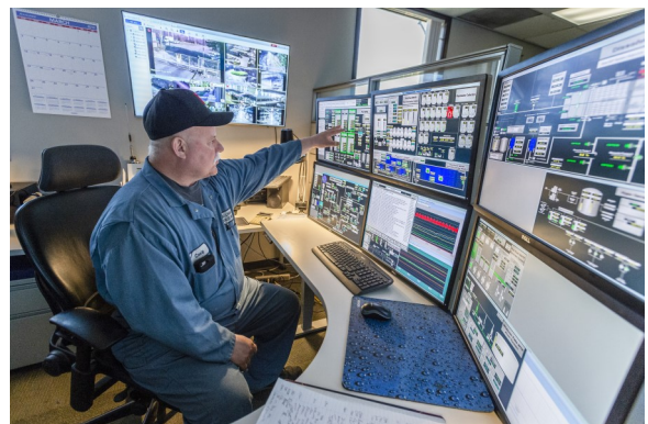
Operator at the Wastewater Treatment Plant controlling the process
