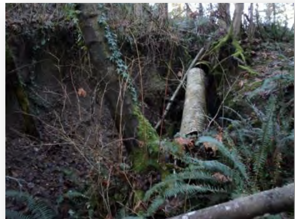
Photo 8. Failing outfall, mass wasting, erosion and incision into road fill north of Lakeway Drive.
