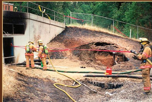
*The blast crater where the pipeline ruptured and the gasoline poured out of the ground. The building on the left of the photo is part of the water treatment plant.*
